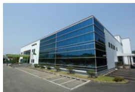
Completed construction of the Daedeok Pharmaceuticals Plant
