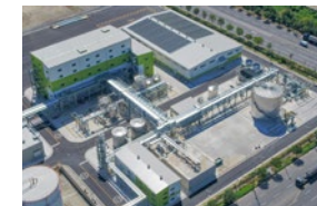
Completed construction of the Gunsan Isosorbide (ISB) Plant for Samyang Innochem
