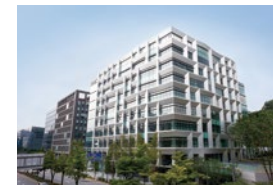
Completed construction of the Samyang Discovery Center
