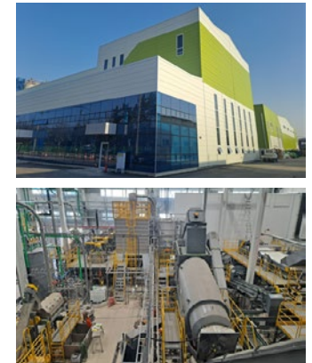
Samyang EcoTech Sihwa Plant
