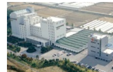
Samyang Corporation Asan Plant
