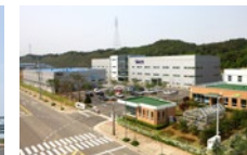
KCI Daesan Plant
