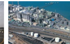
Samnam Petrochemical Yeosu Plant
