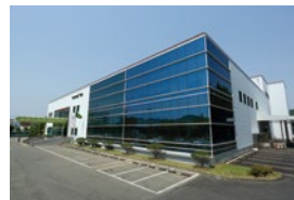
Completed construction of the Daedeok Pharmaceuticals Plant
