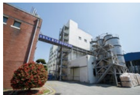
Completed construction of the Jeonju Polyester Plant
