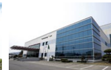
Samyang Holdings MD Plant
